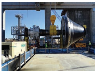
Assembly of the Unit 2 shaft and inner gate barrel on the powerhouse roof at Cannelton.
